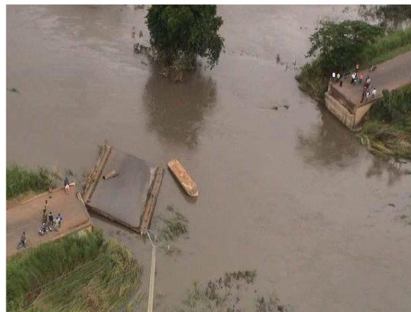
Figure 8: Bridge break on the national road N°1 at AMAKPAPE following the August 2008 floods in Togo (photograph by Togolese National Television, TVT)
