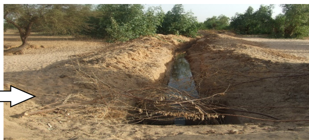
Figure 20: Obstruction of a serving channel with sand transported by Koris water
