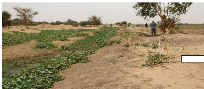
Figure 19: Bottom filling of a drain preventing the circulation of water with sediments brought by the Koris.
